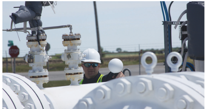
Figure 3: Multiple scans are “stitched” together to generate a contiguous data set. Because of line-of-sight constraints, sites are captured in multiple scans. Scans are then stitched together via a registration process to produce a single contiguous “point cloud.” Registration is achieved by establishing common control points via “registration spheres” that are temporarily deployed across the scan site.
