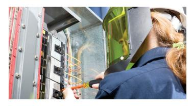
employees with exposure to electric-arc hazards wear protective clothing and other protective equipment with an arc rating greater than or equal to the estimated heat energy whenever that estimate exceeds 2.0 cal/cm2."
